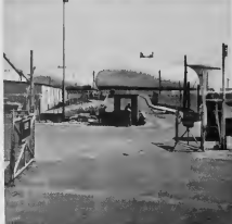
THE CONTROL point of the new road will be at Gate 5, located adjacent to the Mechanical-Garage gate. E PUNTO di control pa e camina nobo lo ta na Porta No. 5, situá cerca di e porta di Mechanical-Garashi.
